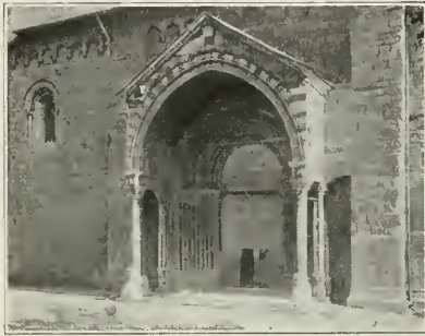
PORCH AND NORTH PORTAL, CATHEDRAL OF EMBRUN
